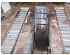
iron with 2x2 slabs in the bottom – does the job, cost next to nowt and pays for itself every time I do an oil change. The garage itself is a DIY affair made from old roof trusses and clad in tongue and groove timber, far enough from the house to allow any amount of noise
